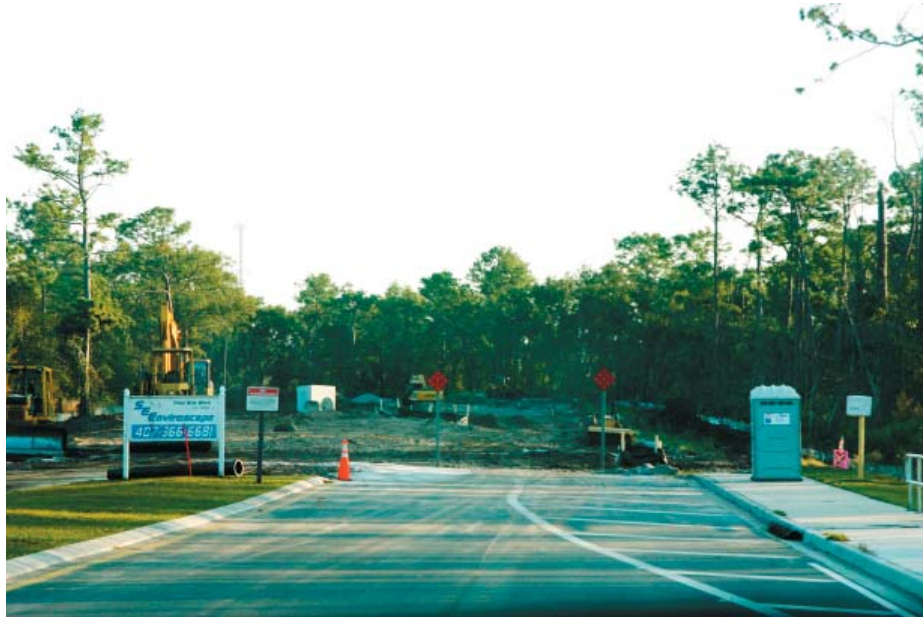
Division Street construction
