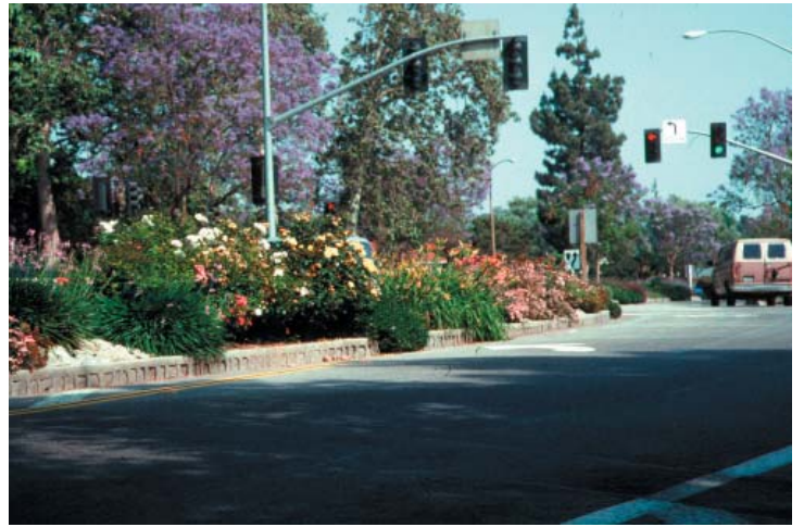
Planted median, Claremont, CA
