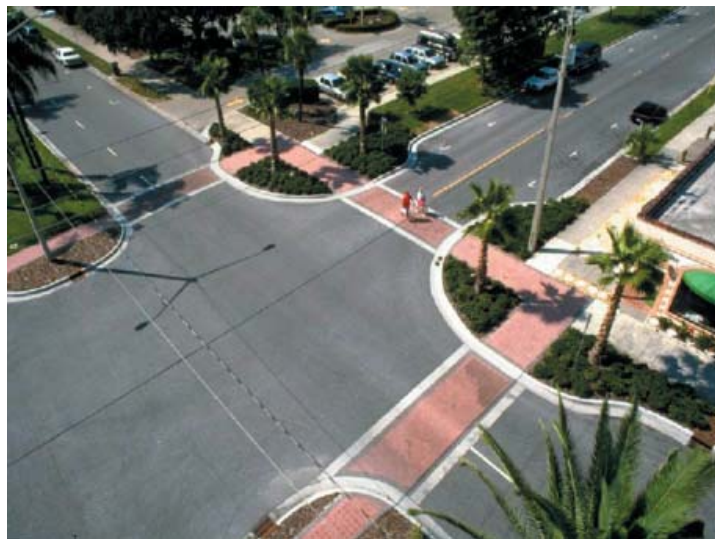
Traffic calmed intersections - Florida
